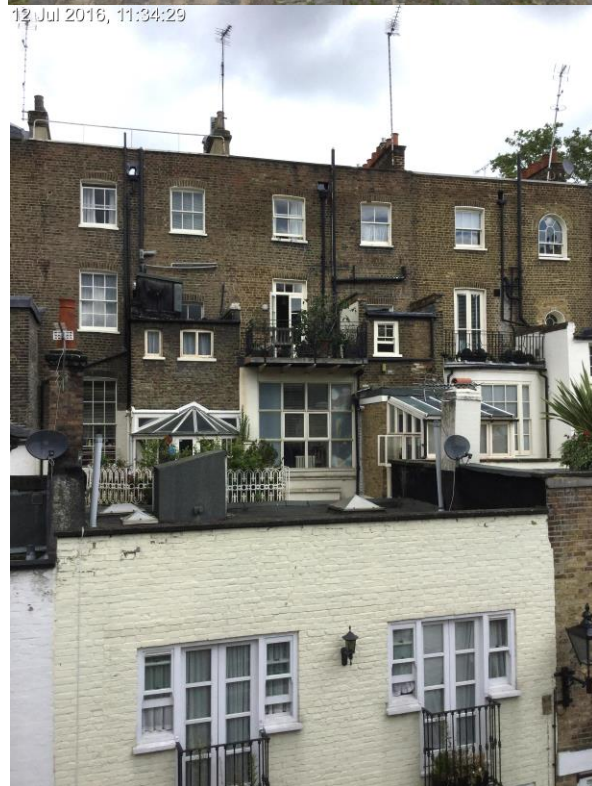
Front elevation of application site (top) and view of roof level (bottom)
